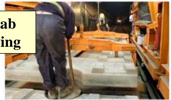
(5) Slab adjusting
