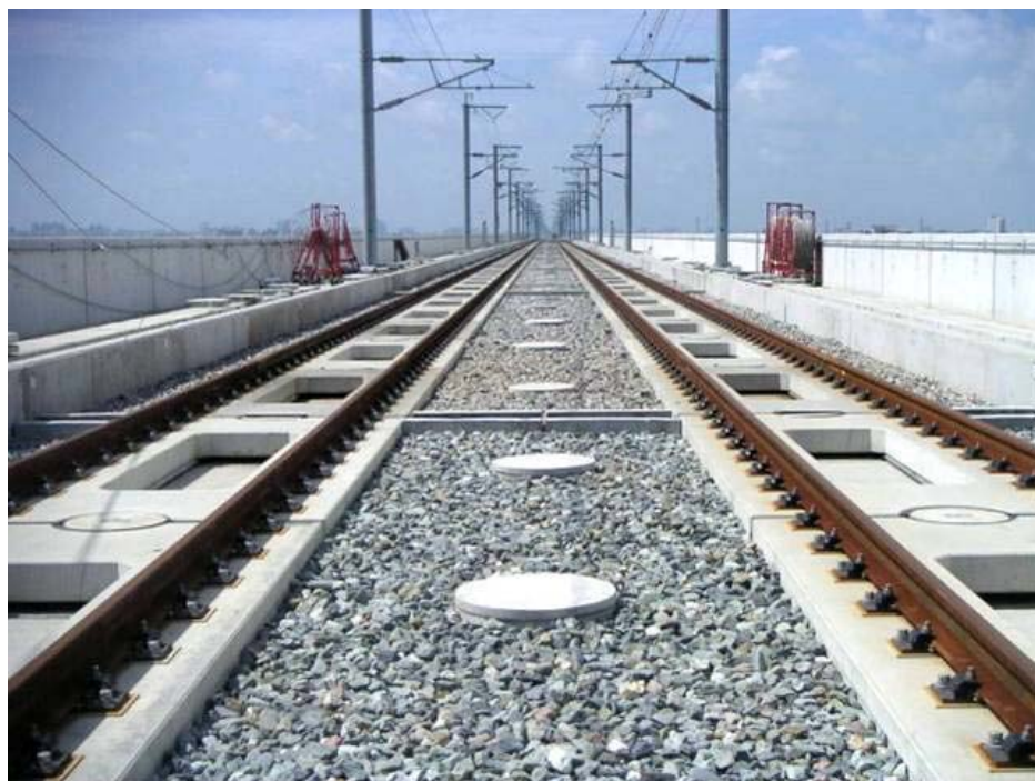
Slab track (Japanese) Standard track structure
