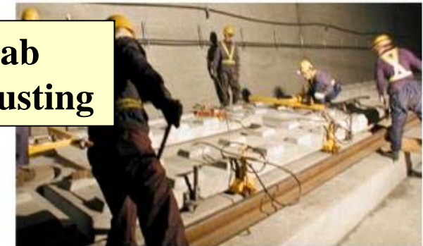
(6) CA-mortar injection
